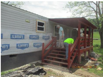
Installing New Windows
