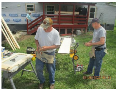
Window Replacement Prep
